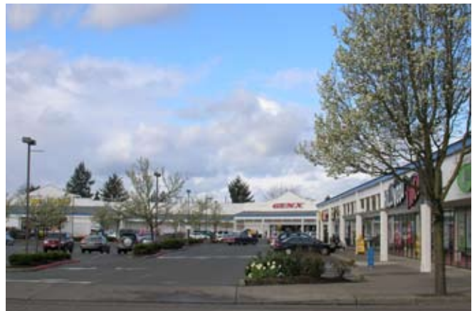
This strip mall, anchored by discount grocer Food4Less and Hollywood Video, is located at the south end of the Corridor study area at the intersection of Powell Boulevard.
