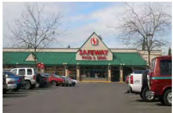
Safeway Anchors the mid-point of the corridor at the intersection of Sandy and Fremont Avenue.
