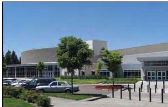
The entrance to Lakeridge High School presents a modern façade of concrete and glass.
