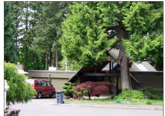
Striking post-and-beam home with an internal orientation, open floor plan and expansive interior glass provides private views of nature.
