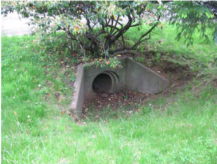
Figure 3.1.6-Mainline overflow culvert at Lori Lane Note the clean culvert inlet
