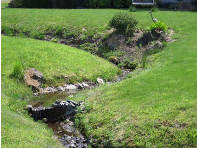
Figure 3.1.5-Mainline creek off 101 north of 7th street Note the clean meandering ditch free of obstructions
