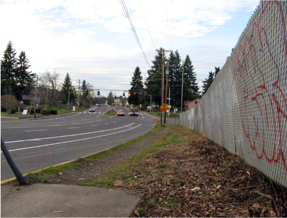
Segment of SE 122 nd Avenue that lacks sidewalks.
