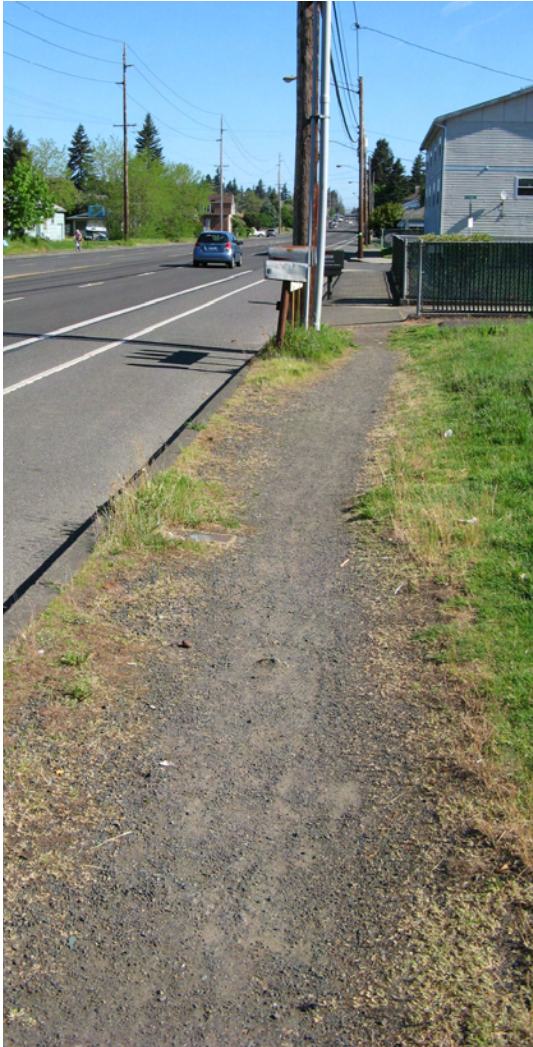
LACK OF SIDEWALKS AND PEDESTRIAN AMENITIES ON 122ND
