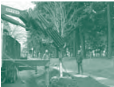
Installing new trees
