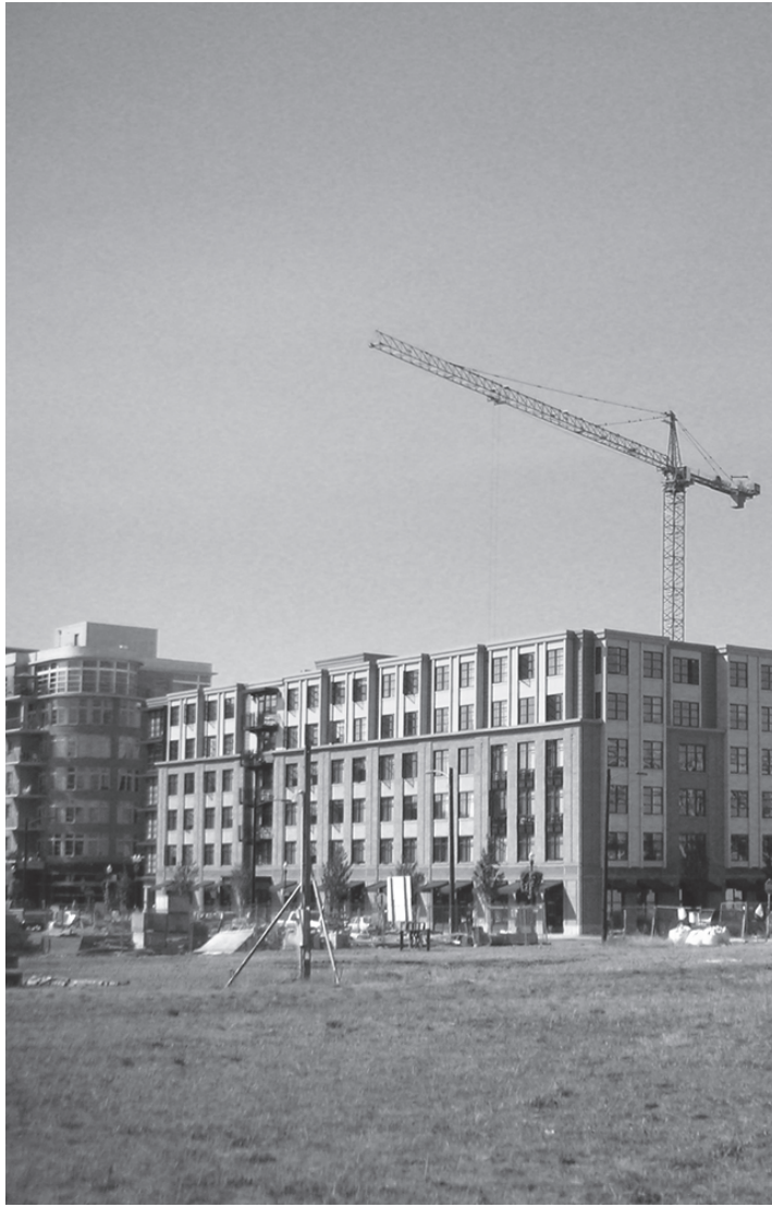
Construction in central Portland's River District
