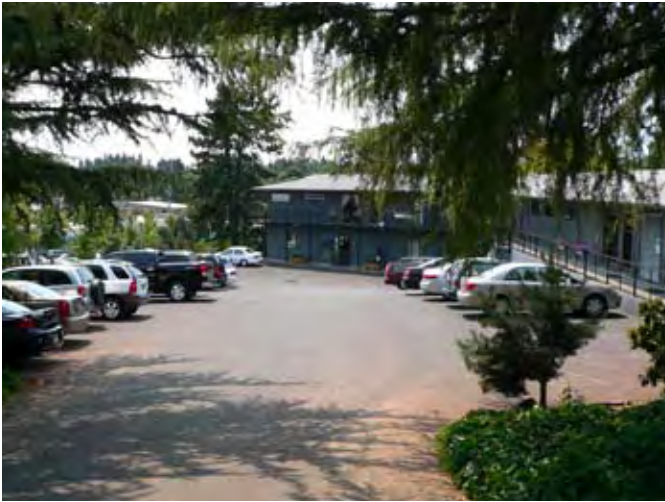
Southwest corner of Sunset and Dewitt View of the medical office building today.
