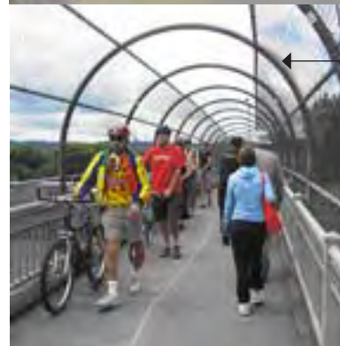
Failing Street Pedestrian Bridge
