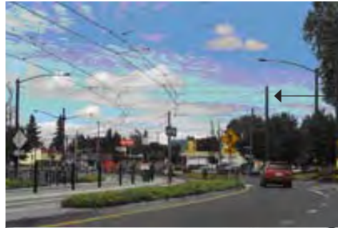
Interstate Ave. between Mason & Prescott
