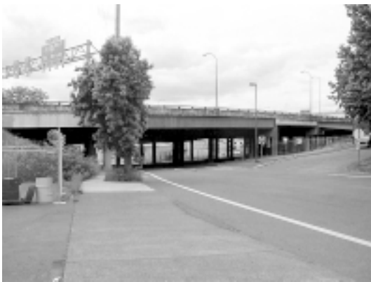
Russell Street at I-5 overpass looking west.
