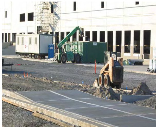
New construction in Rivergate.
