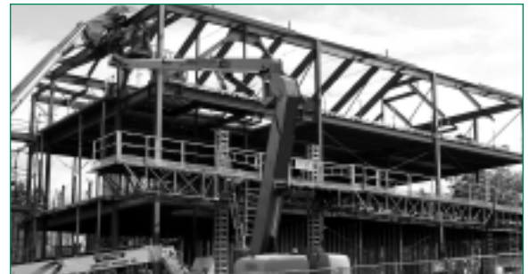
HEDCO building begins to take shape 4/08
