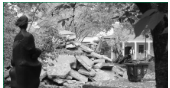
Resurfacing begins as remodeling draws to a close 11/08
