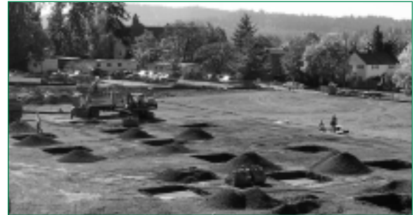
Looking south at footings with trailers in background 10/07
