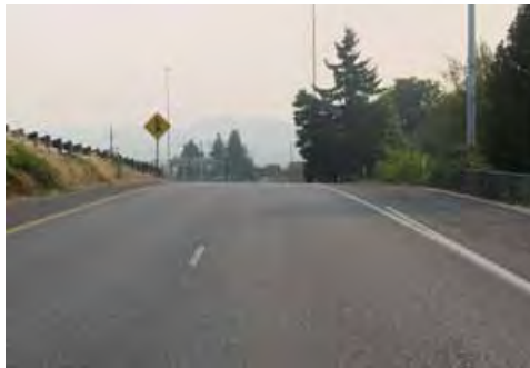
Eastbound Beltline Hwy On-Ramp at River Rd
