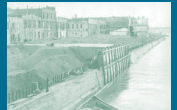
The seawall under construction, 1929
