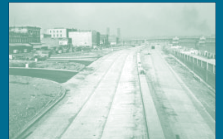
Harbor Drive under construction in the 1940s
