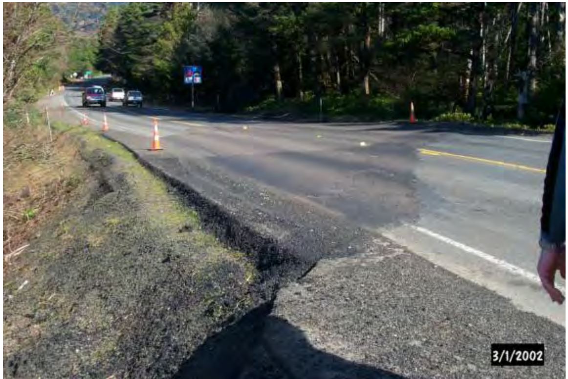
Figure 1: Johnson Creek Landslide on Highway 101
