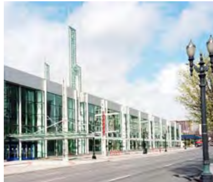
Oregon Convention Center Expansion has made a significant contribution to the character and quality of NE Martin Luther King Jr. Blvd
