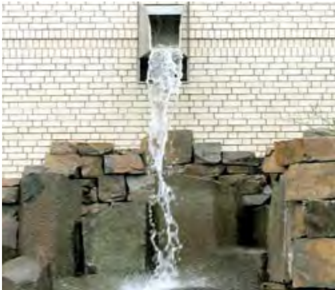
Oregon Convention Center storm water draining into rain garden.
