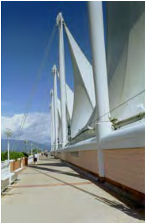
Vancouver Convention Facility, Canada Place
