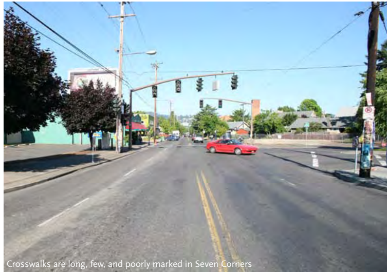
Crosswalks are long, few, and poorly marked in Seven Corners
