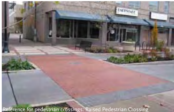
Reference for pedestrian crossings: Raised Pedestrian Crossing
