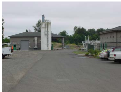
Lime Storage Silo
