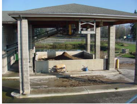
Biosolids Stabilization Area
