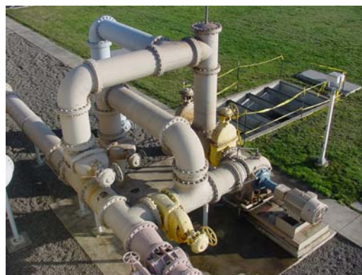
Outdoor Process Piping
