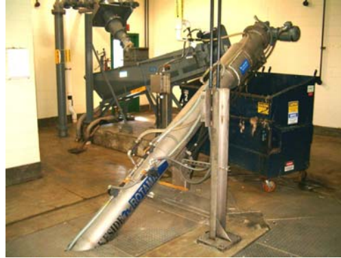
Influent Screen and Grit Washer
