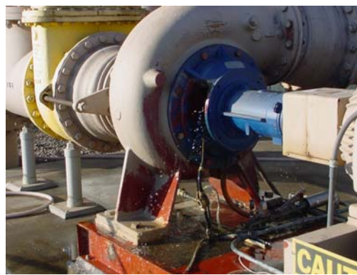
Reactor Mixing Pump
