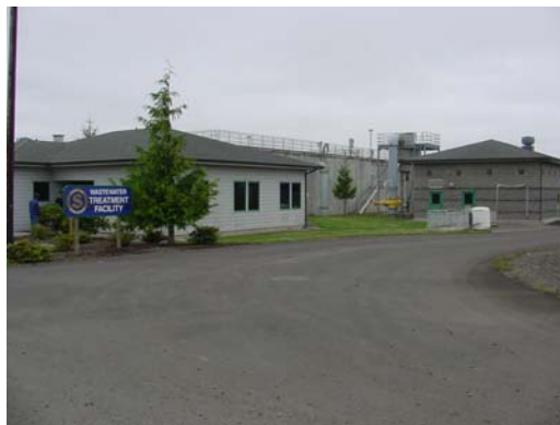
Existing Treatment Plant
