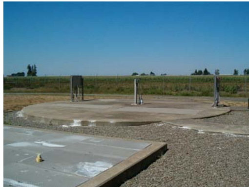
Influent Pump Station
