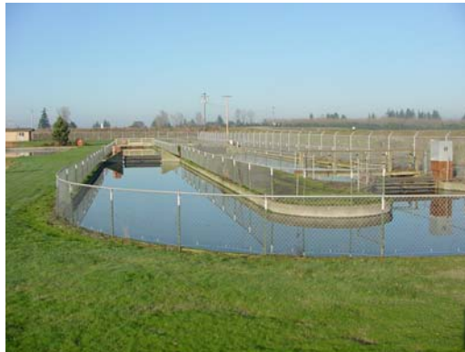
Abandoned Oxidation Ditch
