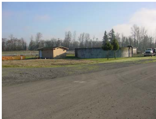
Aerated Sludge Storage Tank
