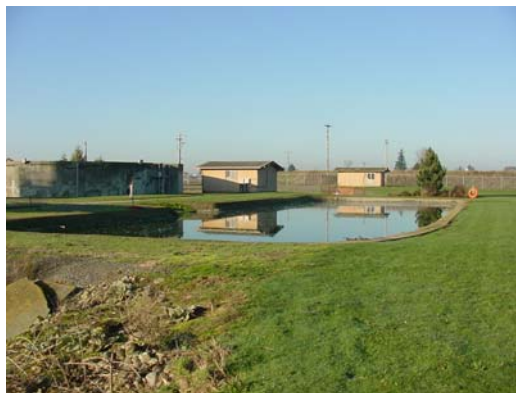
Liquid Sludge Storage Pond
