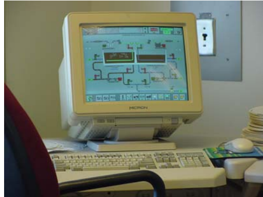
Computer Monitoring and Control System
