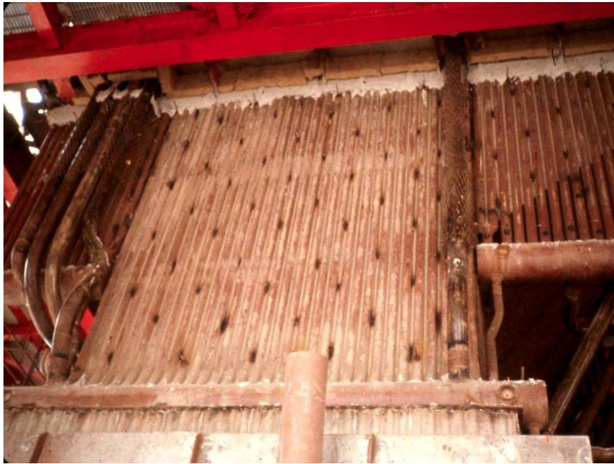
Figure 1- Waterwall Furnace Section 2
