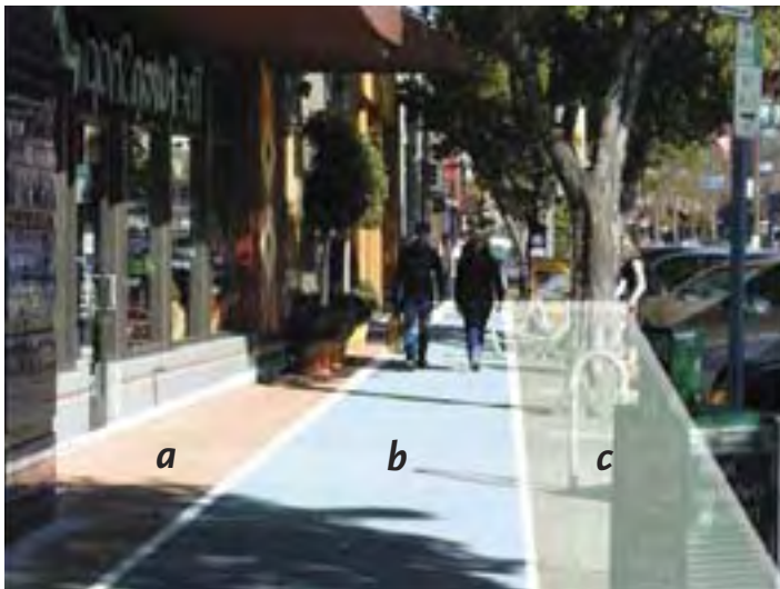
SIDEWALK DESIGN—SHATTUCK AVENUE, BERKELEY, CALIFORNIA a) frontage zone: canopy & merchandise display; b) through pedestrian zone; c) furnishings zone
