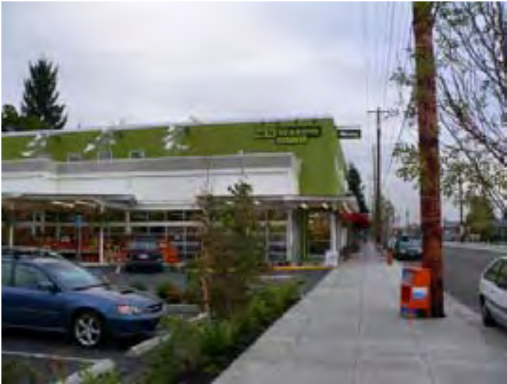
RELOCATED PARKING Parking located to the side of auto-oriented retail
