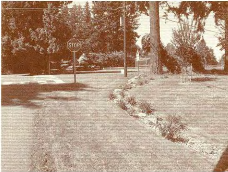
This curbless neighborhood street in Lake Oswego infiltrates and conveys stormwater runoff in a landscaped infiltration trench. A sidewalk could be constructed in the grassy area.
