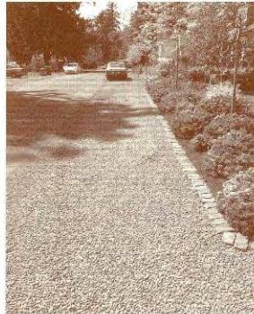
Crushed gravel allows stormwater infiltration in the parking area of this residential street.
