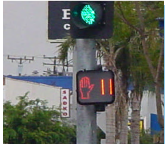
Pedestrian crossing countdown signal
