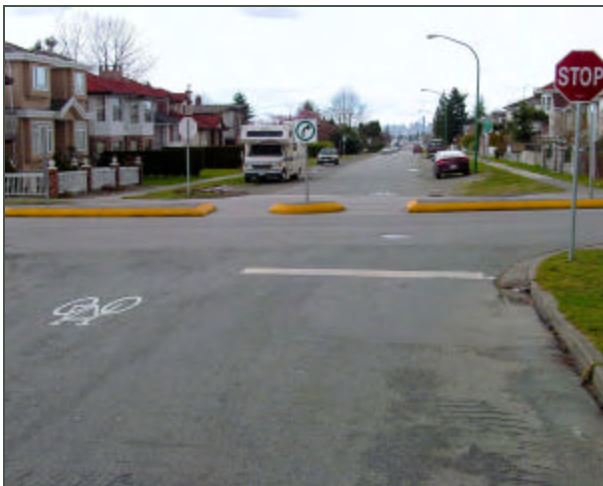
Traffic diverters: median island (left) and bike/ped only refuge on NE 16 th and Tillamook in Portland (right).
