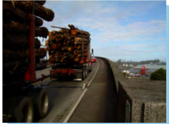
Yaquina Bay Bridge sidewalk with truck traffic
