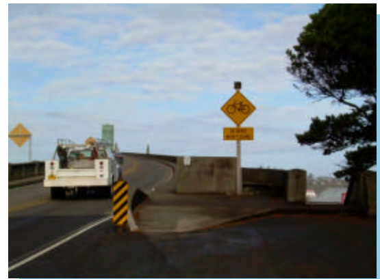
Existing signage for crossing Yaquina Bay Bridge
