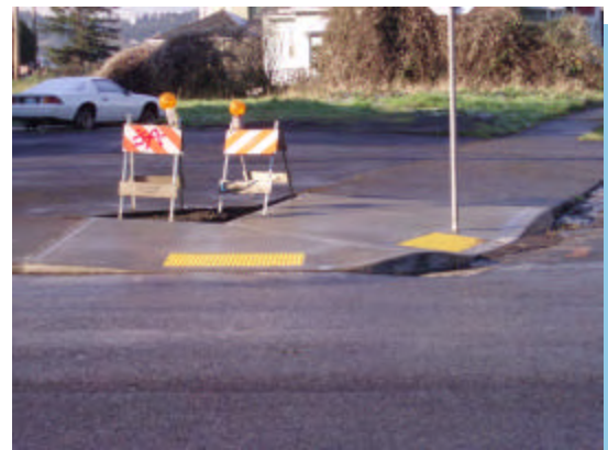
Dual curb ramps with detectable warning strips
