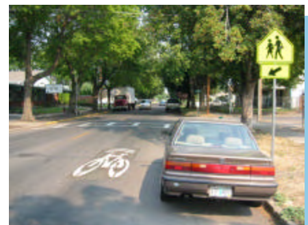
Sharrow placement on a local street
