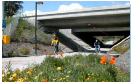
Type 4 Grade-Separated Undercrossing
