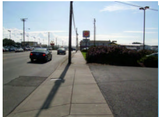
Sidewalk on U.S. 101 near 15th Street
