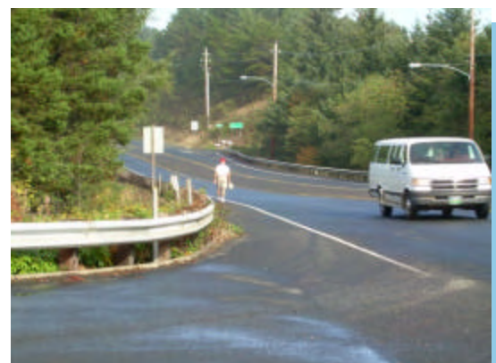
Debris in the bikeway on U.S. 101
