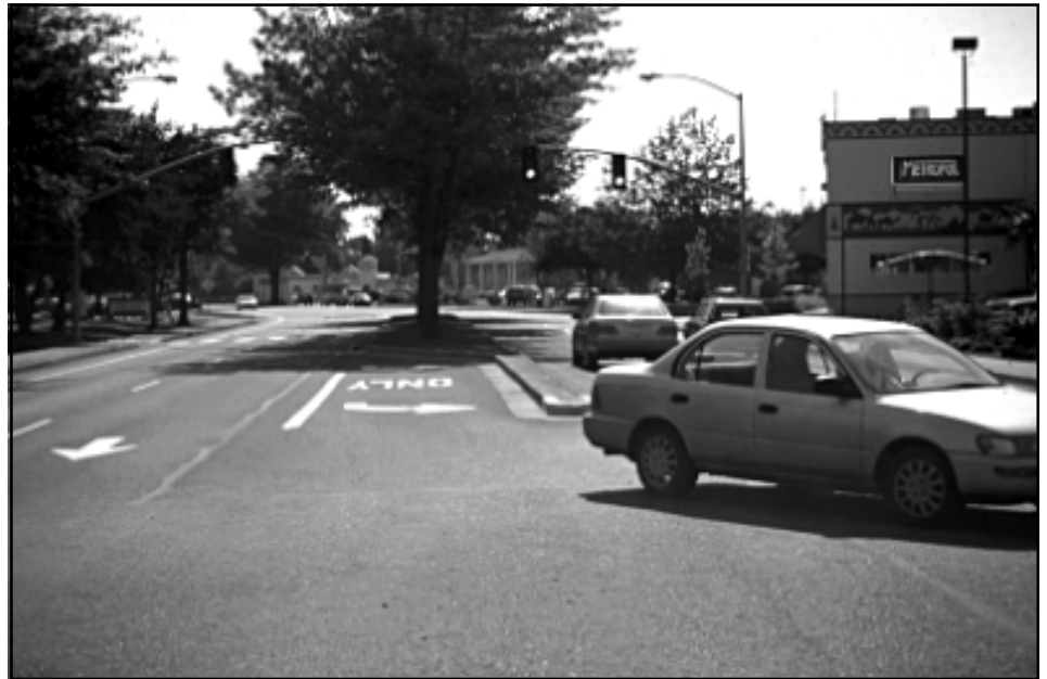
Trees planted within median islands reduce the perceived width of the street.
