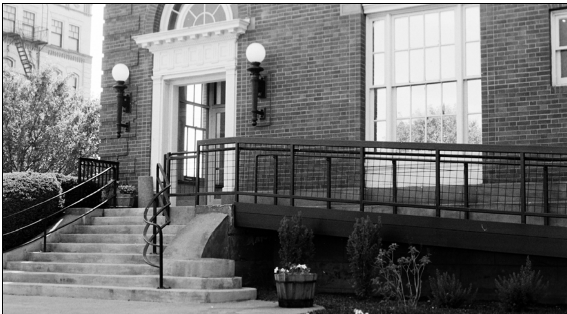
La Grande City Hall – the historic integrity of the north and west entries has been maintained. The ramp and railing have been added to the secondary elevation of the building at the southwest corner.
