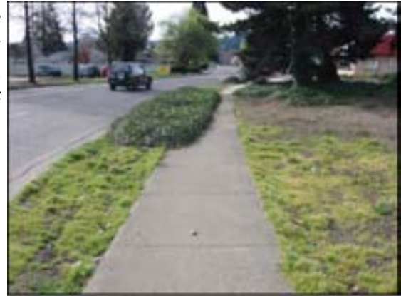
Figure 6. Vegetation Encroaching on Sidewalk
