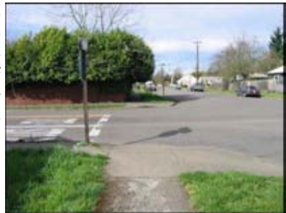
Figure 7. Vegetation Restricting Vertical Clear Distance
