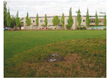
Drainage Problems on Softball Field
