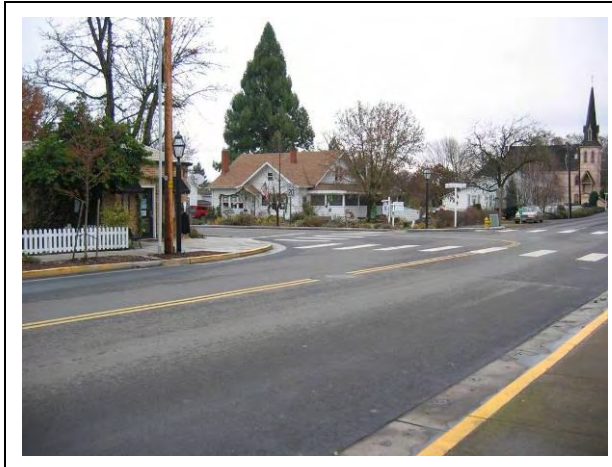
OR 238 (5th Street) @ California Street: Looking northeast through intersection from southwest corner.
