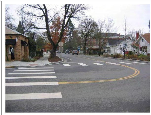
OR 238 (5th Street) @ California Street: Looking north across intersection from southwest corner.
