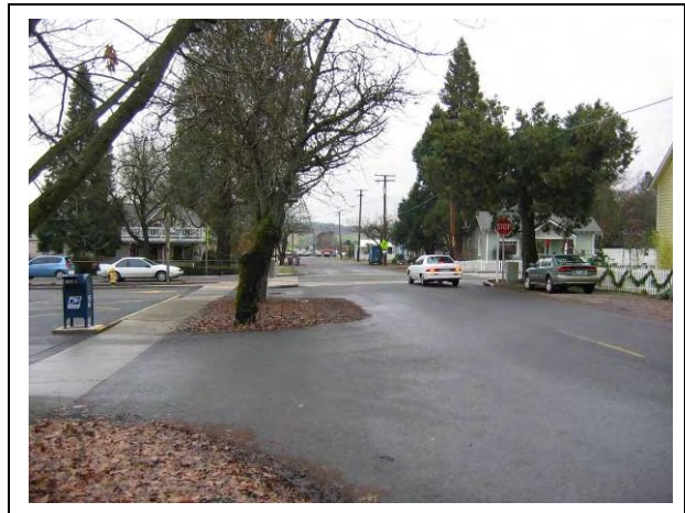
OR 238 (5th Street) @ E Street: Looking east through intersection along north side of E Street.
