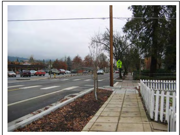
OR 238 (5th Street) @ E Street: Looking north through intersection along east side of 5th Street. Jville08.jpg
