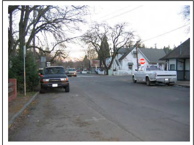
Oregon Street @ C Street: Looking east along C Street through intersection at Oregon Street.
