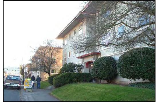
Streetcar-Era apartment building with 18' front setback, located on the Hawthorne Boulevard main street.
