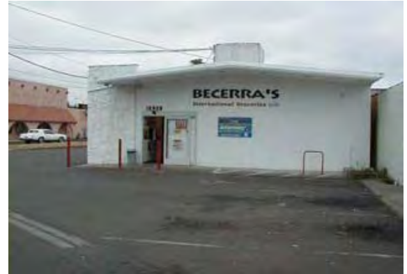
Poor Building Orientation
