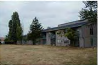
Daret Property- view northwest
