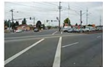
Stark crossing Burnside- view west
