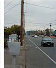
Stark- view east
