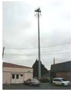
Stark St- view to north
