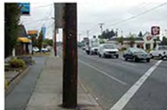
Stark St @ Burnside- view east
