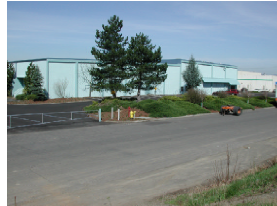
Example of Site in Need of Sidewalks and Curbs
