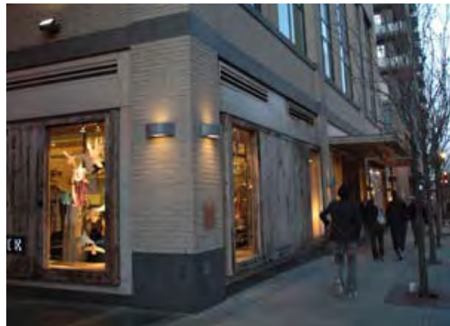
Fig. B.10.c.2 salvaged material integrated into the ground level facade in a prominent manner
