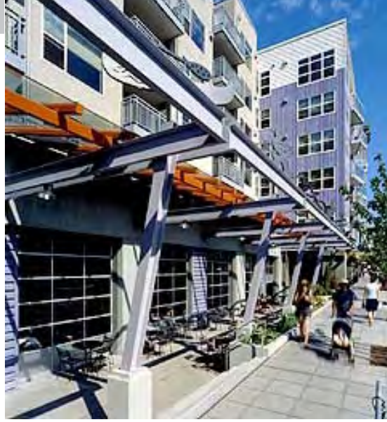
Fig. B.3.c.2 colorful, expressive ground-level facade elements help animate the street
