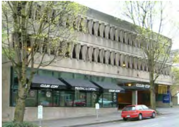
Fig. A.4.C.1 Parking garage structure lined by retail uses.
