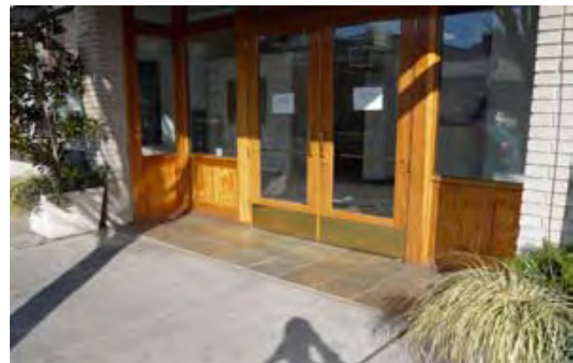
Fig. B.6.d.4 (1) 2 ft recessed doorway with tile accent at entry
