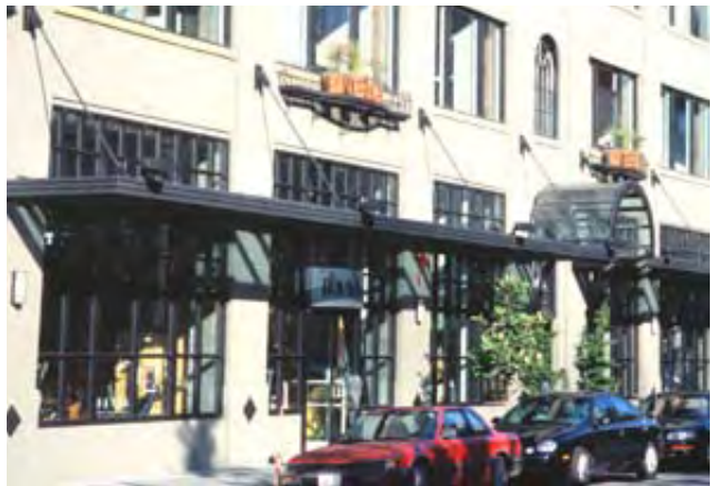
Fig. B.3.c.3 medallions, seasonal planting, recessed entry, pedestrian signage all integrated into the building facade
