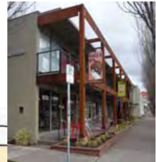
Fig. E.3 (2) Cor-ten steel portico adds to the three-dimensional quality of this commercial building
