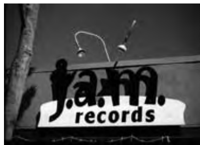
Fig. B.4.c.1 (2) lights shielded toward sign
