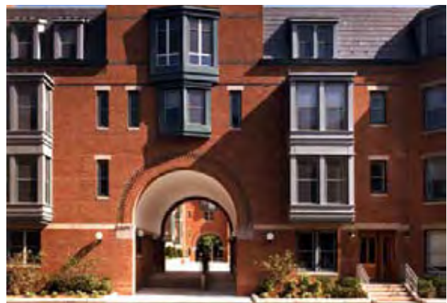
Fig. B.6.c.4 (2) arched entry
