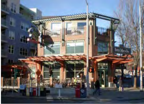
Fig. B.3.c.1 a robust array of building components and ornamental detail
