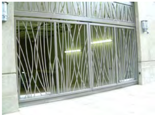
Fig. A.4.c.4 parking structure with decorative metal screening
