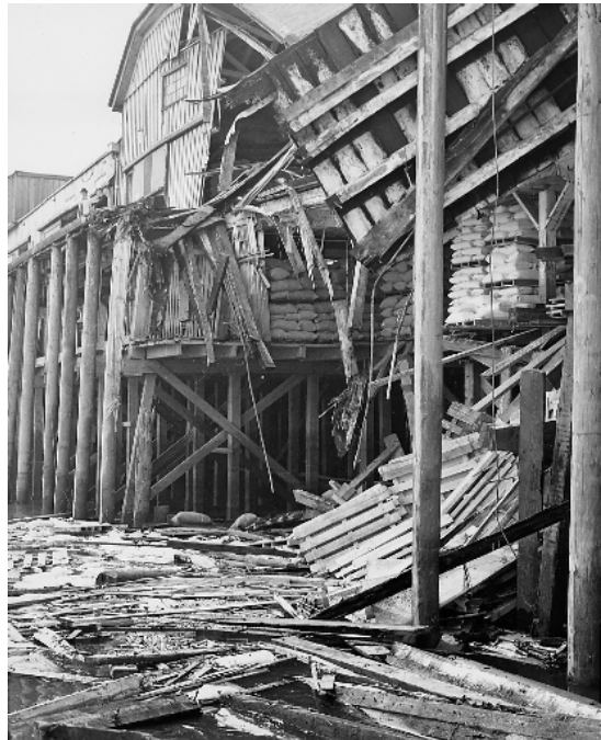
Collision damage from the Aegean Mariner, 1965
