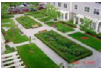
Courtyard infiltration basin at Buckman Heights Apts.
