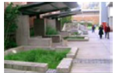
Stormwater planters to underground rainwater harvesting system
