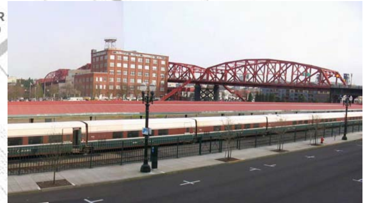
VIEW OVER RAILROAD
