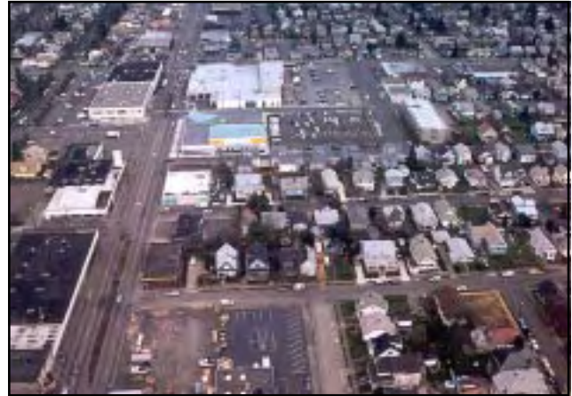
The Multnomah County building at the upper left and Marco Machine Works in the center occupy a significant portion of the project area.
