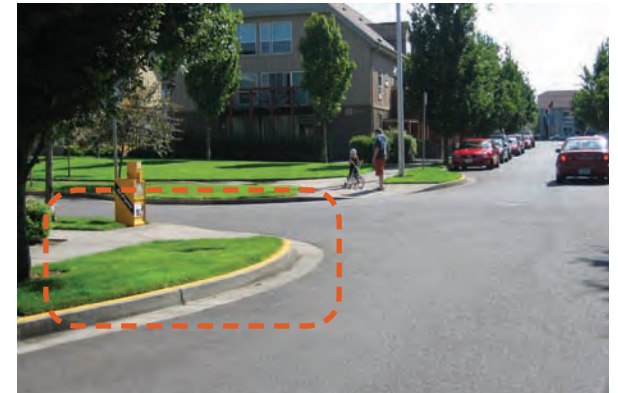
Existing curb extensions in Gateway provide traffic calming and improved pedestrian connectivity. The GGSMMP proposes combining these and other techniques to improve pedestrian connectivity, safety and storm water quality.
