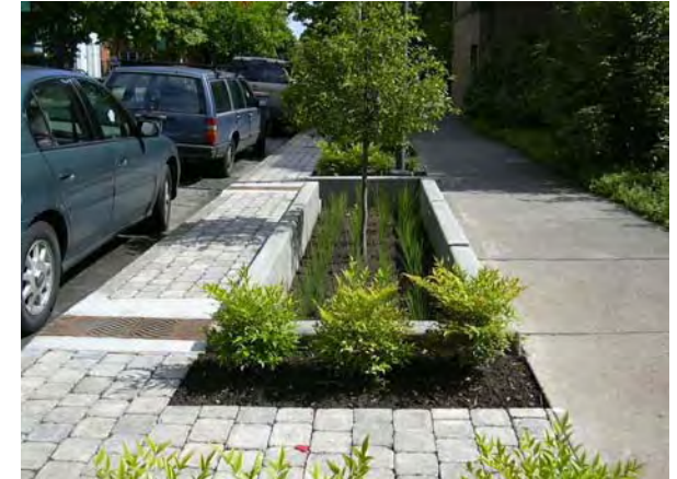
Stormwater planters at SW 12th Ave. create a unique identity with aesthetic treatment of stormwater.
