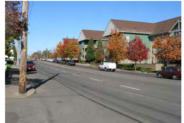
The existing NE 102nd Avenue ROW has sufficient width to allow a future retrofit that includes a new median. NE 99th Avenue may also have sufficient width for such a median.
