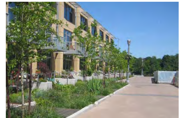
Pennoyer Street in the South Waterfront District utilizes stormwater swales, porous pavers and an asymmetrical centerline to slow vehicles.
