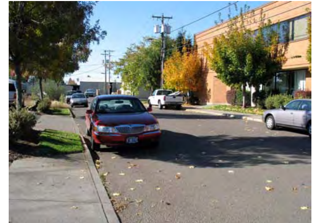
An existing ROW with the potential for application of the 63' Green Street Typology. Newer building in photo shows potential urban character of this area and an example of half-street improvements as this street is converted to green infrastructure incrementally.
