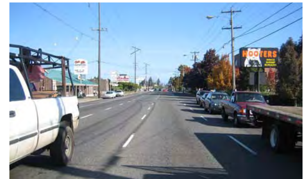
SE Stark Street--Arterial featuring 4 vehicular lanes, on-street parking on both sides and a bicycle lane
