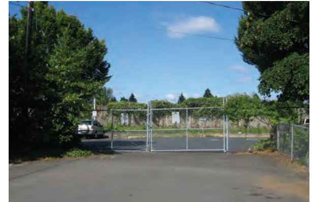
Some future street ROWs are currently blocked or non-existent (NE Flanders Street at NE 99th)
