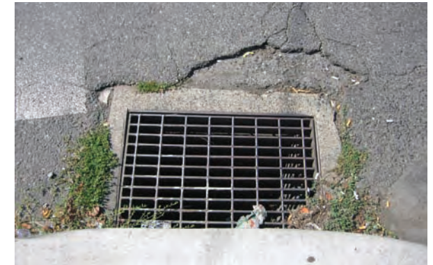
Half of the sumps are connected to sedimentation manholes and half are connected directly to catch basins.
