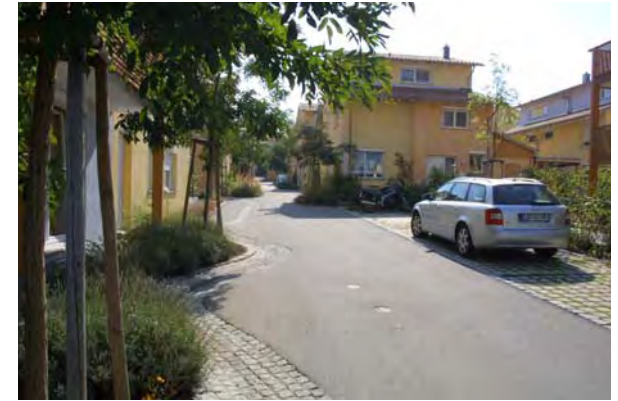
A curbless residential 'woonerf' street in Stuttgart, Germany that incorporates stormwater swales and grass pavers in the parking zone.
