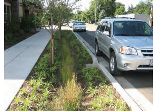
Existing stormwater management in the Gateway District ROW demonstrating a vegetated street swale.
