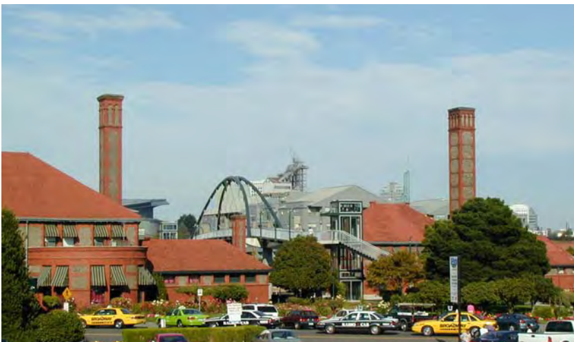
Union Station Pedestrian Bridge
