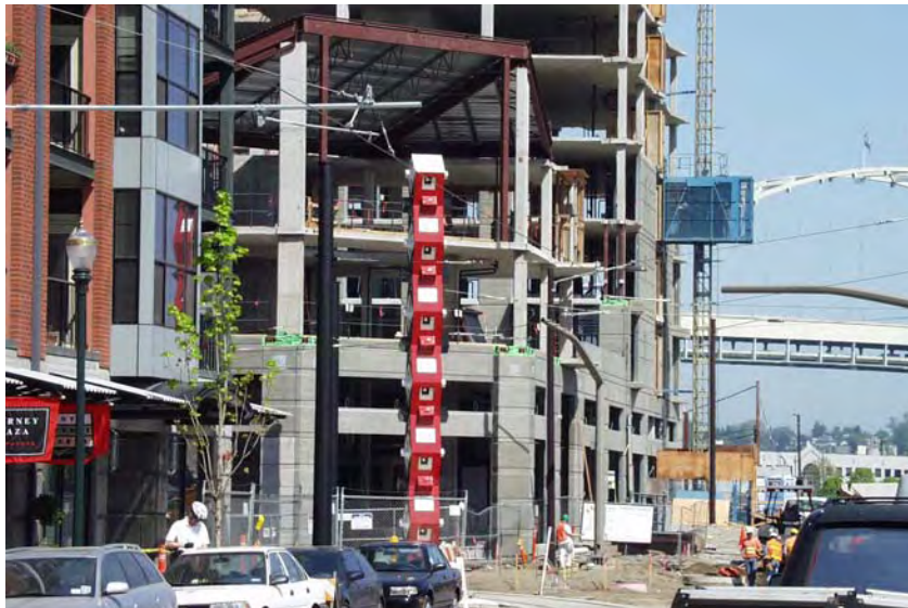
Works in Progress at NW 11th Ave. and Kearney St., June, 2001
