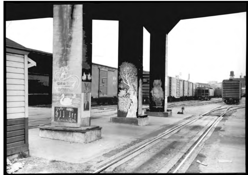
Lovejoy Columns (Photograph by Larry Smith, 1954. Courtesy of Thomas Robinson)
