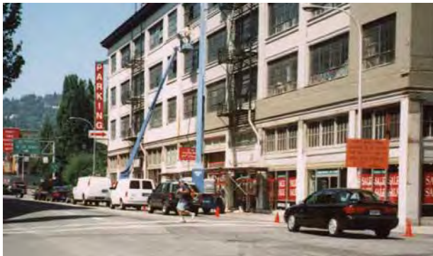
NW 13 TH AVENUE/BURNSIDE STREET
