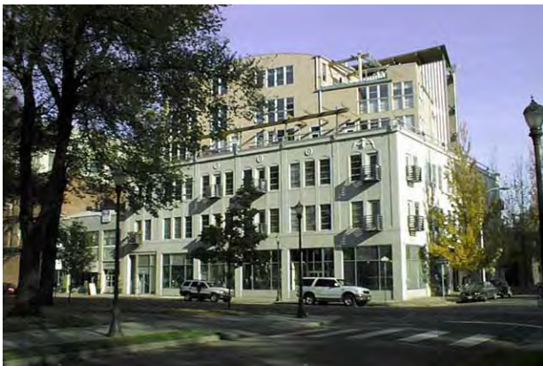
725 FLANDERS BUILDING (NW 8TH AVE./FLANDERS ST.)
