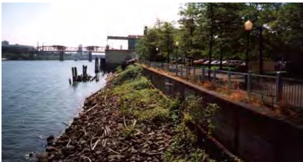
FREMONT PLACE LOOKING SOUTH
