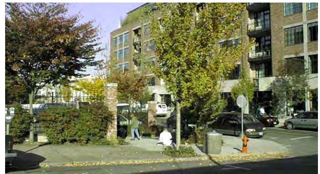
MCKENZIE LOFTS (NW 12 TH AVE./FLANDERS STREET)
