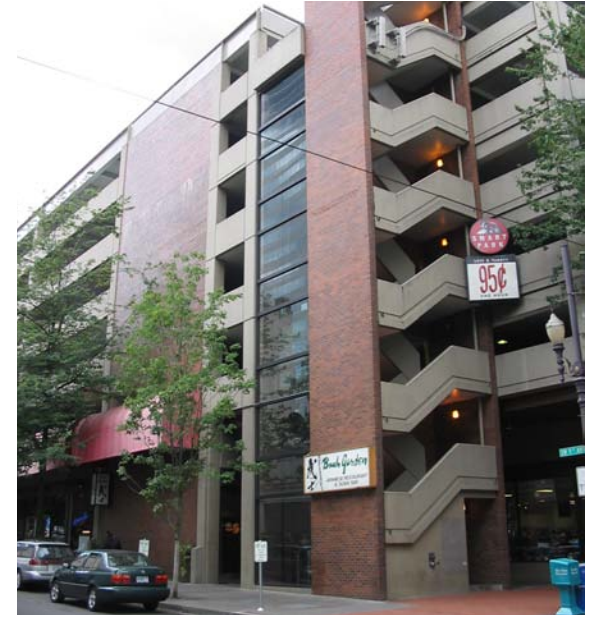
corner stair and elevator
