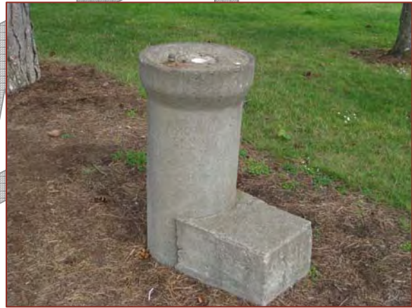
Figure 5. Damaged, non-ADA compliant drinking fountain
