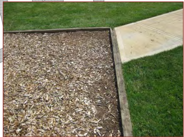
Figure 14. Playground access requires ramp for ADA compliance
