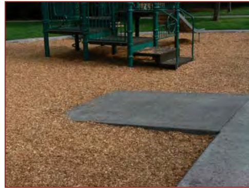
Figure 35. Example of ADA-compliant ramp into play area
