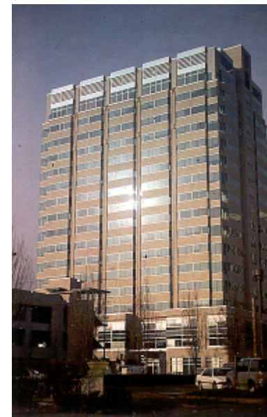
Liberty Centre office tower.
