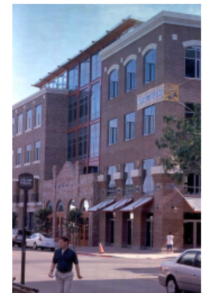
Mixed use residential condominium, ground floor commercial/retail and flex office space in San Diego, California.
