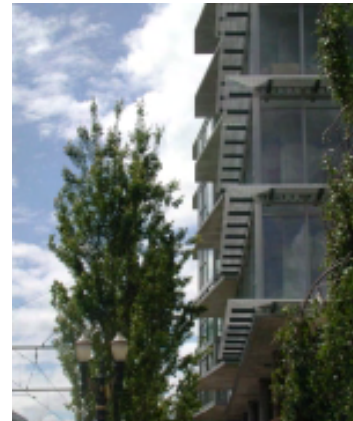
Cascadian condominiums Phase I nearing completion, 2001.
