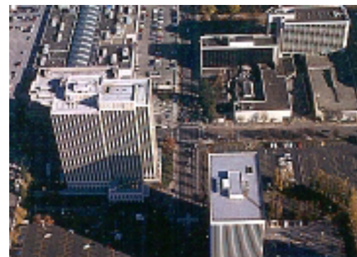
Parking lots are often vacant after hours because of insufficient District activities. Parking primarily serves employees and events at the OCC and Rose Quarter.
