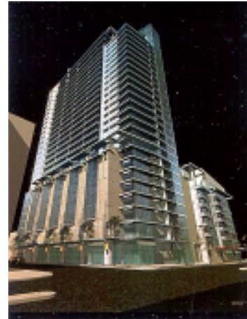
Cascadian condominiums at Northeast Grand and Holladay. The first phase, an 8-story block, began construction in Fall 2000.
