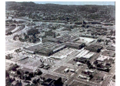
Lloyd Center opened in 1960. The Sheraton Hotel is south of the shopping center overlooking Holladay Park.
