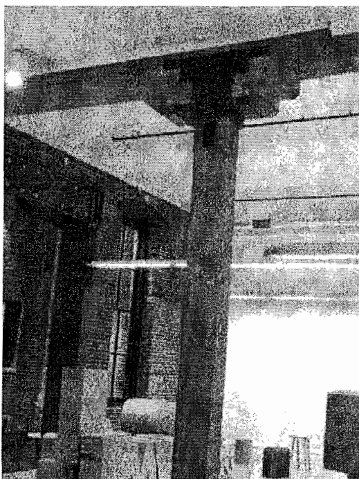
Figure 4.6 Reconstructed and reinforced capitals of the Skidmore building that were damaged when the south façade was removed for the construction of the Burnside Bridge in 1926. Photo by author, 2008.
