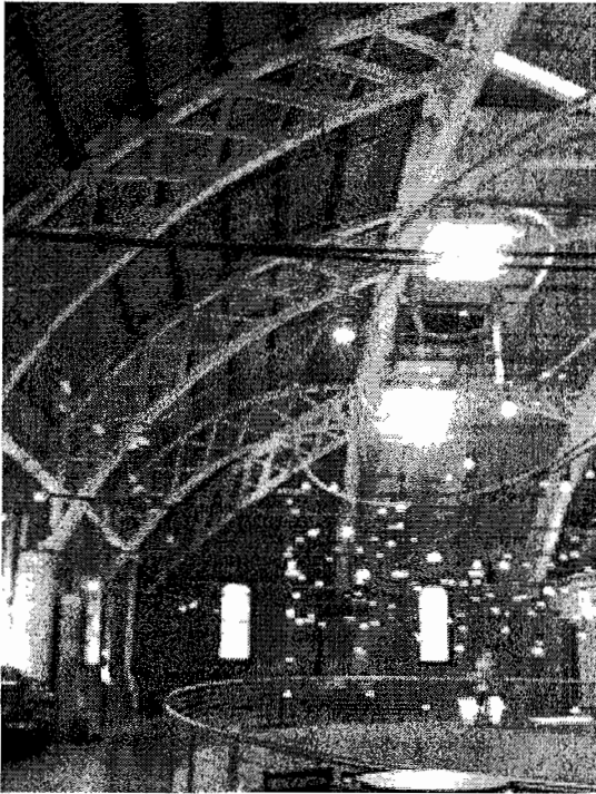
Figure 5.4 As a character defining feature of the Annex, the unique bowstring truss system was left exposed. Interior design draws visitors attention to the structural system with the lighting design on the mezzanine of the lobby. The photo by author
