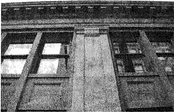
Figure 3.4 Sandstone, double hung windows, and dentil cornice of the south façade. Removing multiple layers of paint revealed a sandstone veneer that was preserved and treated for protection against graffiti. Photo by author, 2009.
