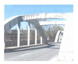
**Figure 18:** Rogue River (Caveman) Bridge, 1931, illustrating vertical and horizontal scoring in the concrete *Source:* Author
