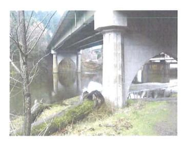
**Figure 39:** Reused piers from the original Eagle Creek Bridge constructed in 1936 *Source:* Author
