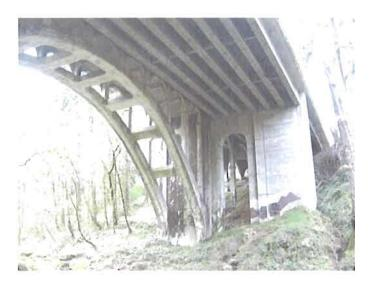
**Figure 46:** Historically incompatible deck widening from 1983 at Sucker Creek (Oswego) Bridge in Lake Oswego, 1920
