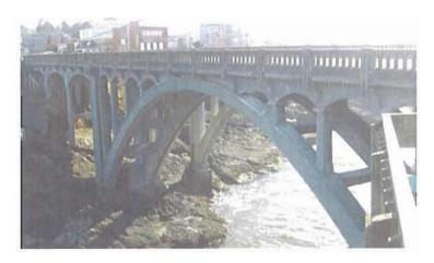
**Figure 45:** Historically compatible 1940 deck widening at Depoe Bay Bridge on US 101, 1927
