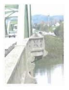
Figure 11: South Umpqua River (Winston) Bridge, 1934, illustrating deck widening for inclusion of pedestrian walkway Source: Author
