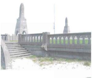
**Figure 37:** Reuse of entrance pylons, towers, and staircase at new Alsea Bay Bridge at Waldport, 1991 *Source:* Author
