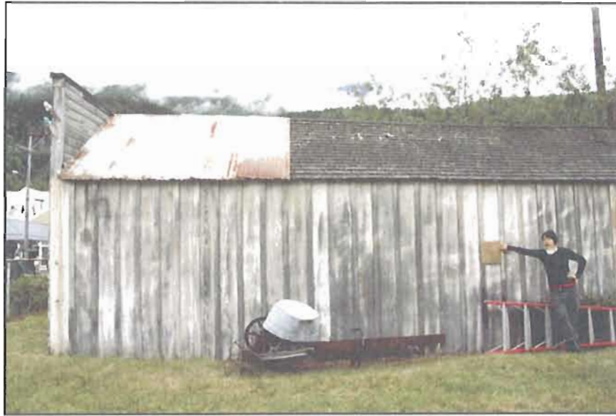
Figure 17. East elevation with board and batten siding. Source: National Park Service/Alaska Regional Office, July 2008.
