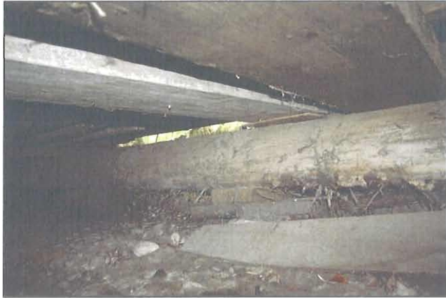
Figure 15. Log foundation along east wall of section A-1. Source: National Park Service/Alaska Regional Office, The Jeff. Smith's Parlor Museum Historic Structures Report, 2008.
