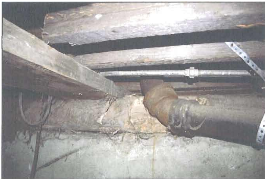
Figure 16. Log foundation along west wall of section A-2. Source: National Park Service/Alaska Regional Office, July 2008.
