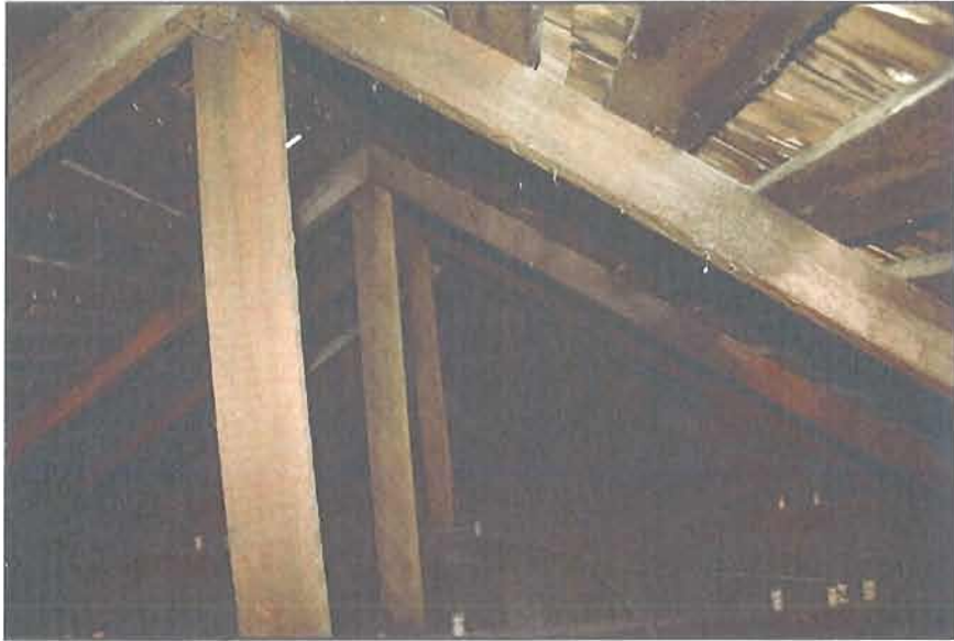
Figure 21. Attic A-1 rafters at ridgeline. Source: National Park Service/Alaska Regional Office, July 2008.
