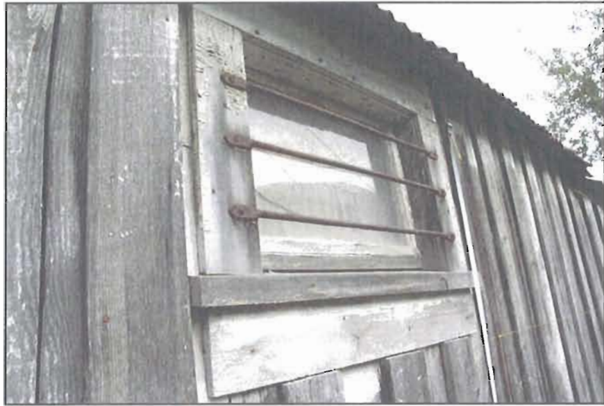
Figure 19. Window and metal bars on east elevation. Source: National Park Service/Alaska Regional Office, July 2008.
