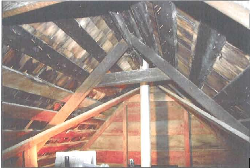
Figure 22. Attic B ridgeboard, rafters and collar ties. Source: National Park Service/Alaska Regional Office, July 2008.
