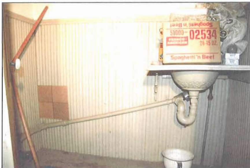
Figure 27. Sink and plumbing in bathroom. Source: National Park Service/Alaska Regional Office, July 2008.
