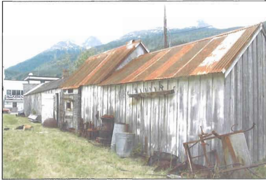
Figure 20. Metal gable roof of section B and C southwest elevation. Source: National Park Service/Alaska Regional Office, July 2008.
