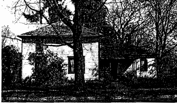
Figure 44. 2110 Trade Street Southeast, Built 1905. Frank Shultz is listed at this address in 1930.
