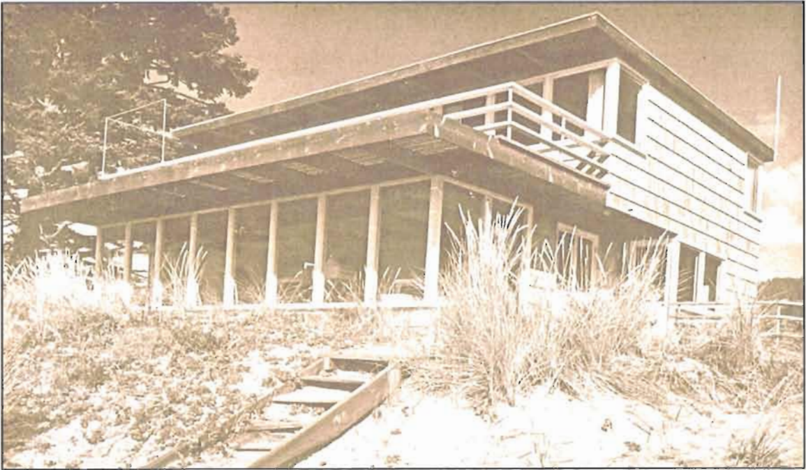
Figure 26: The Harry Blair House. Designed by James Van Evera Bailey. This house was featured in the 1952 Sunset Ideas for Cabins and Beach Houses . Photo courtesy of Visual Resources Collection, Architecture & Allied Arts Library, Building Oregon: Architecture of Oregon & the Pacific Northwest Collection. Copyright 2008, University of Oregon Libraries. All rights reserved.
