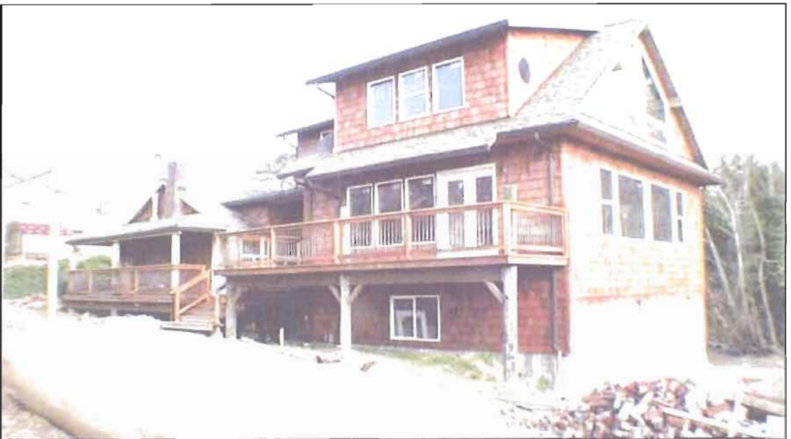
Figure 46: Completed addition to the Umi House. Tillamook County Tax Records Photo, 2006. http://www.co.tillamook.or.us/gov/A&T/public/
