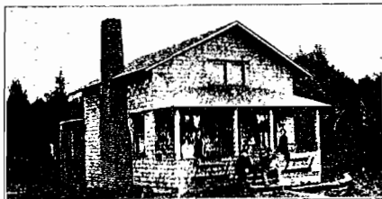
Cottage at Manzanita Beach
