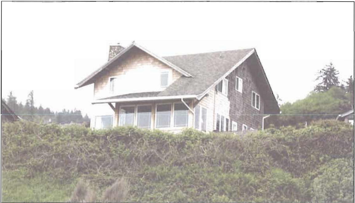
Figure 41: A. E. Doyle's Churchill cottage, Neahkahnie Beach. Note new shingles on front portion of the house. The house also has vinyl windows and a composite roof, both non-historic replacements to this 1913 house. Photo by author.
