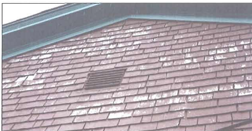
Figure 42: Paint chipping from shingles on the south facade of 1920s house. The house was painted approximately three years before this picture was taken. Photo by author.
