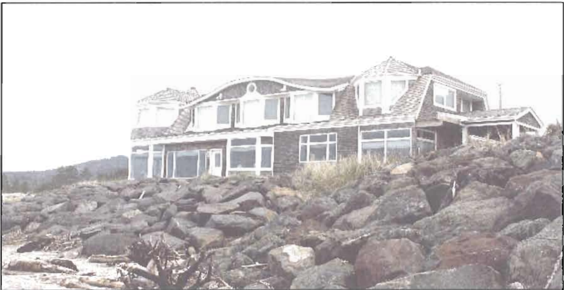
Figure 39: David Beach House and bolder riprap wall. Note the change in the landscape and the growth of the riprap wall. This photo was taken in April of 2009 by the author.
