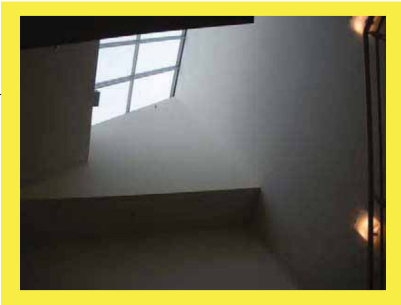
lights add daylight in stairwells
