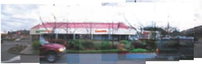
Looking South onto Site
