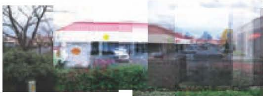
Looking East onto Site
