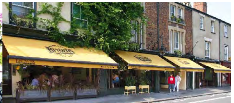
continuous overhead weather protection
