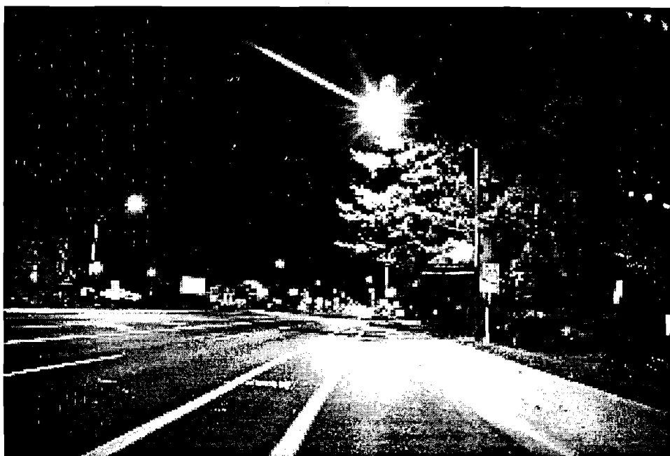
Figure 3-1. On higher speed urban roads, low-level tungsten lights on high-angle cobra mounts provide even lighting to the entire roadway.
