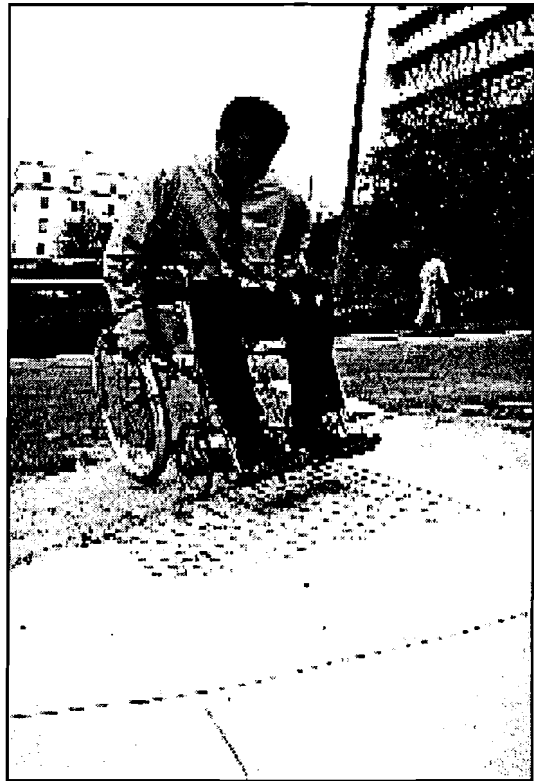
Figure 5-3. A pavement grinding project left an exaggerated lip at this curb cut.
