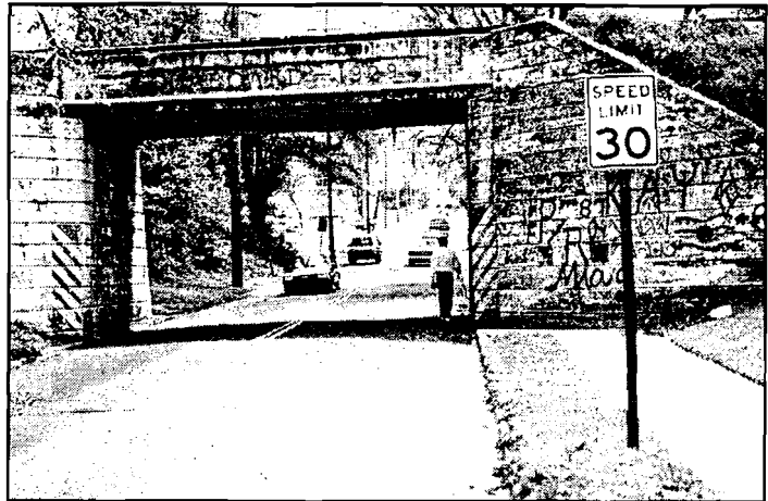
Figure 1-2. Along many streets, sidewalks are either discontinuous or nonexistent.
