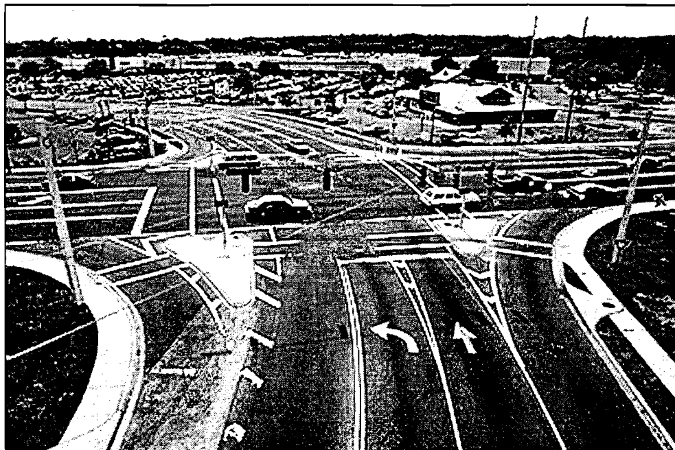
Figure 11-6. Right-turn slip lanes, where the right-turning traffic must yield before entering the roadway, are a safer alternative for pedestrians than double right-turn lanes.
