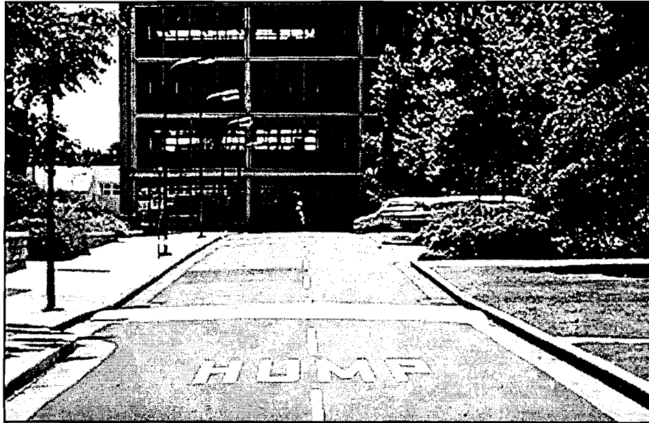
Figure 15-6. Speed humps are intended to reduce traffic speeds to 32 to 40 km (20 to 25 miles) per hour.
