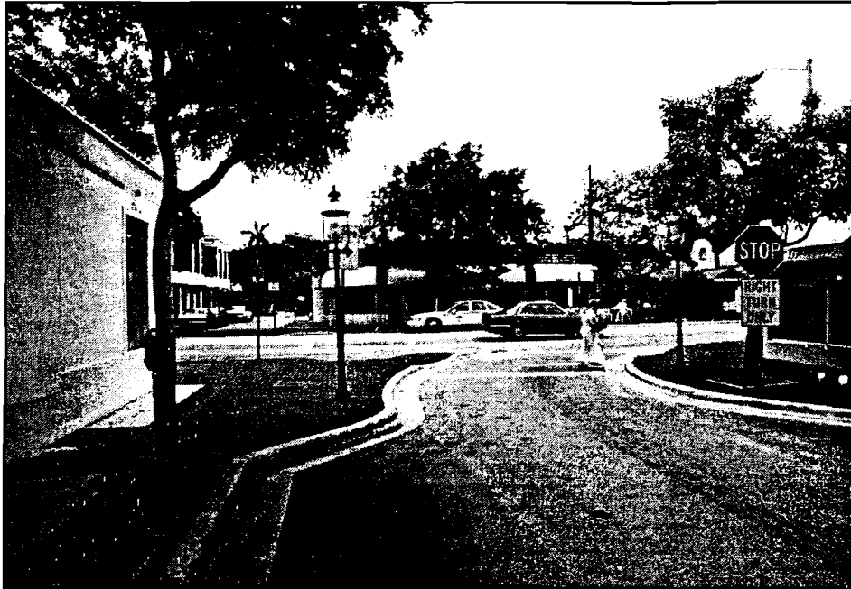
Figure 15-5. A choker (curb bulb) used on a one-way residential street.
