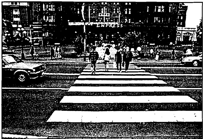
Figure 9-5. High-visibility markings such as longitudinal lines may be used in crosswalks for increased emphasis.
