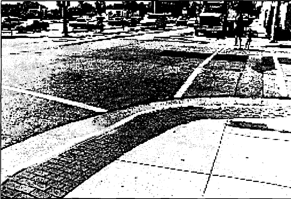
Figure 5-2. Curb cuts are the single most important design consideration for persons in wheelchairs.
